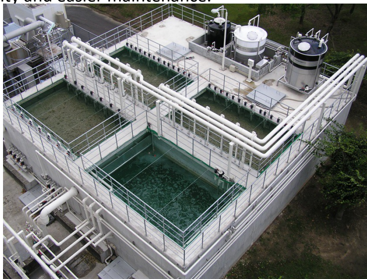
MBR Facility Overview
